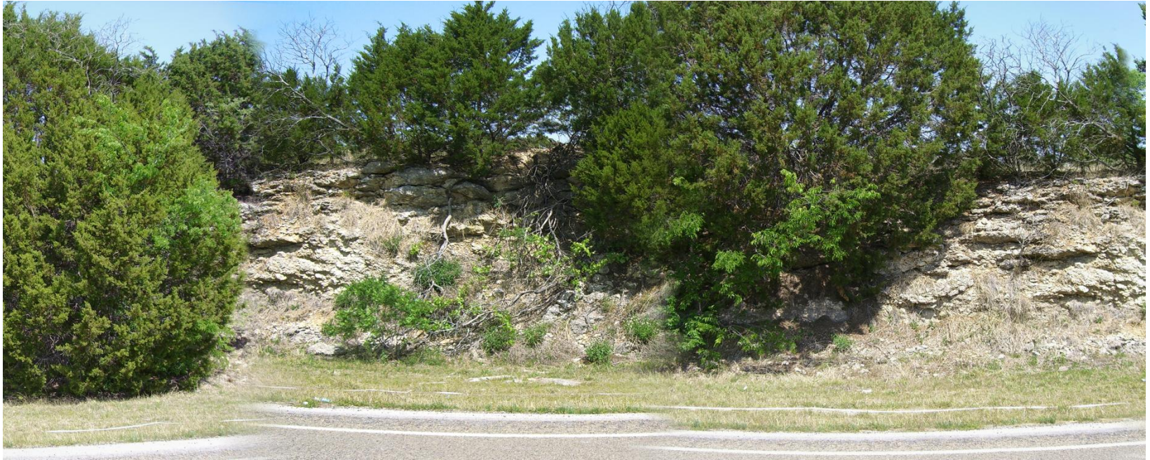
Figure A18. Composite panoramic 8 of 10: of Mosheim-2 between columns 7 and 8.
