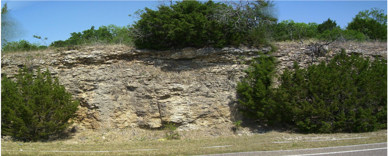
Figure A13. Composite panoramic 3of 10: Mosheim-2 between columns 3 and 4.
